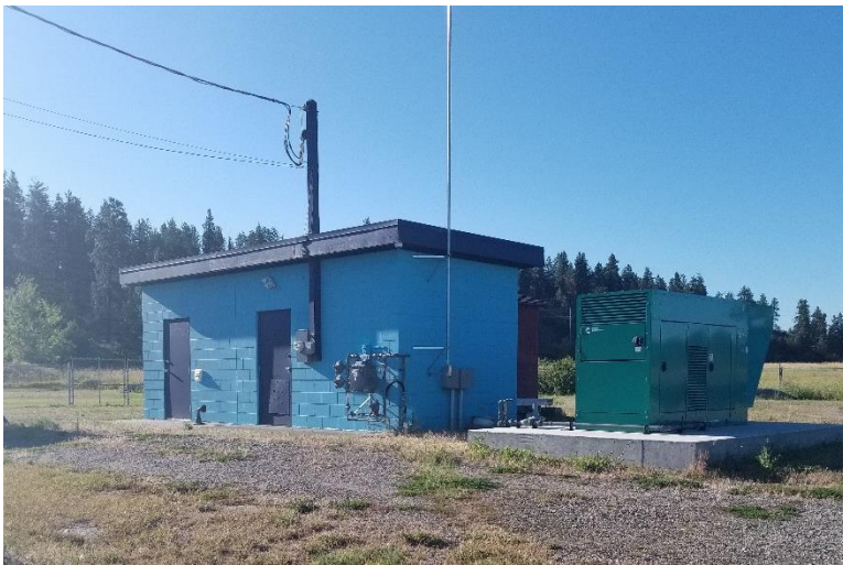
Lodge Road Pump House
